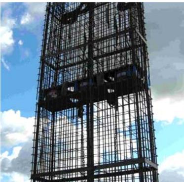
Cage Placement with O-Cell assembly
