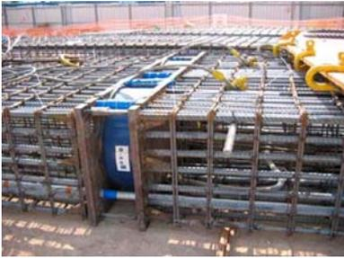
O-cells are installed within the barrette reinforcement
