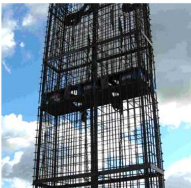
Cage Placement with O-Cell assembly
