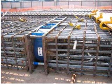
O-cells are installed within the barrette reinforcement
